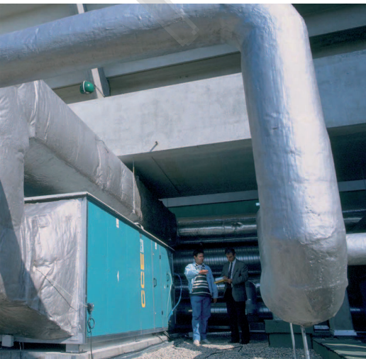
Circulating pumps for building management
