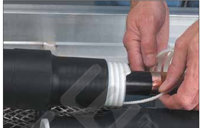
2. Position splice and unwind core
