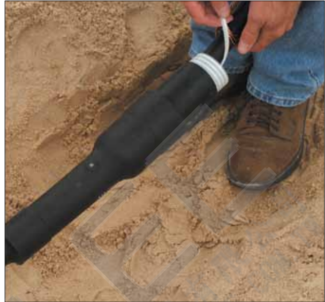
2. Position splice and unwind core
